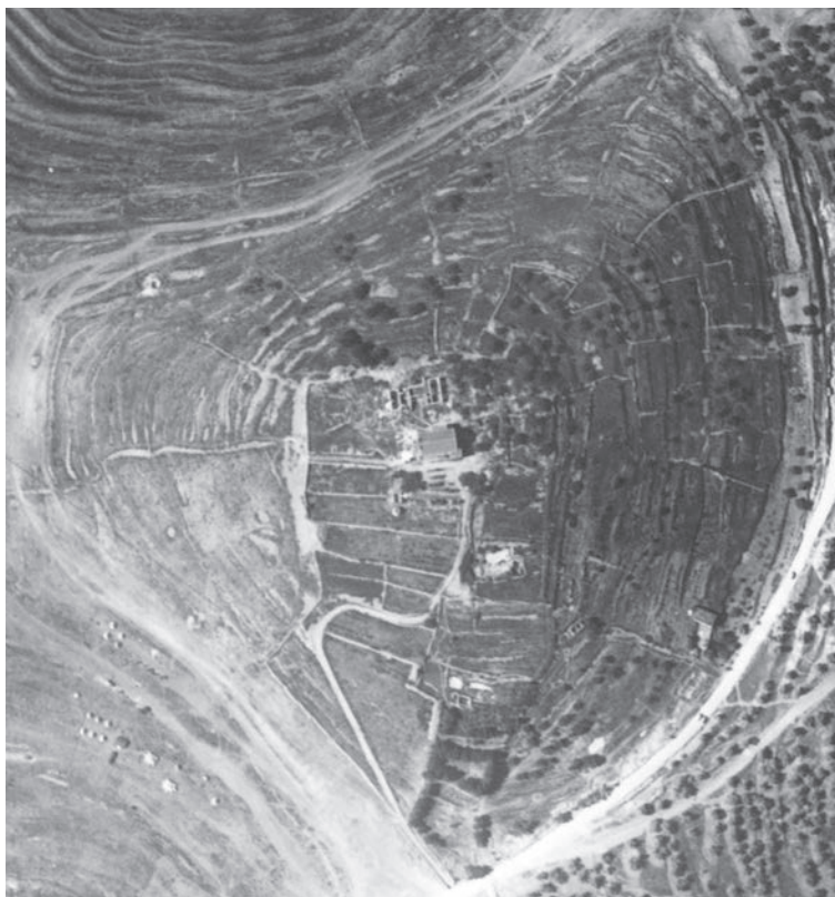
Fig. 1.8: Aerial view of the site, taken by the Bavarian air force in 1918, looking north; note the large western and eastern terraces; the modern building is the convent; to its north are the foundations of the northern sector of the hostel (the church was not built yet)
