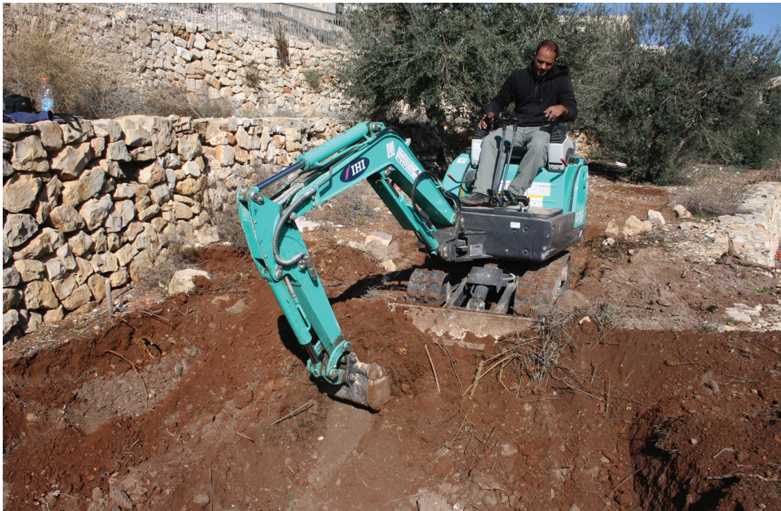
Figure 1.3: Removal of concrete terraces using mechanical tools (February 2013, photo by author).
